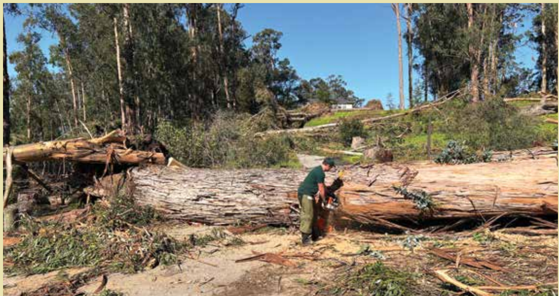
Park rangers are working hard to clear the mess left behind. Trees came down across roads, trails, bridges and power lines.
