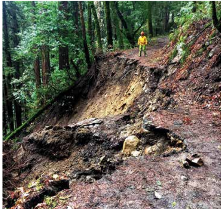
Alambique Trail in Wunderlich Park was washed away by a mudslide.
